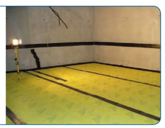
PRODUCT CODE M5 STUD DEPTH 3mm ROLL WIDTH 2m ROLL LENGTH 30m WEIGHT 38kg
