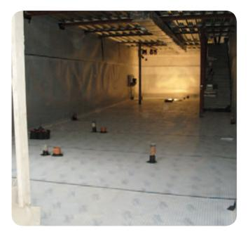
When the waterpoofing fails, Newton System 500 is the perfect remedial solution. Many designers are recognising the advantages of including Newton System 500 to the Type B waterproof structure because of the possibility of leaks through the construction joints. In doing so they have already included what would be their preferred remedial system within the initial waterproofing design.
