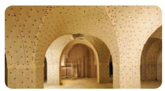
The four images show Newton System 500 applied to the subterranean vaults of the Grade One Listed Royal Courts of Justice in Central London. The images show just how flexible and accommodating the Newton membrane, in this case Newton 508 Mesh, can be. The detailing to the vaults was very intricate and had to be completed by the Newton NSBC Contractor to a very high standard ready for plastering.
