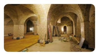
With Newton System 500 it is possible in some circumstances to install a system that is completely reversible, which can be removed at a later date. English, Scottish and Welsh Heritage often stipulate that the waterproofing is both reversible and causes little or no damage to listed buildings.
