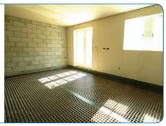
PRODUCT CODE M4 & M13 STUD DEPTH 20mm ROLL WIDTH 2m ROLL LENGTH 20m & 10m WEIGHT 36.30kg & 18.15kg
