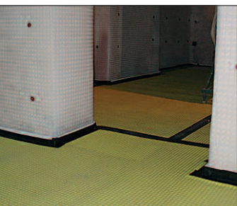
Above: Newton 300 used as a flooring membrane when part of Newton waterproofing system.
