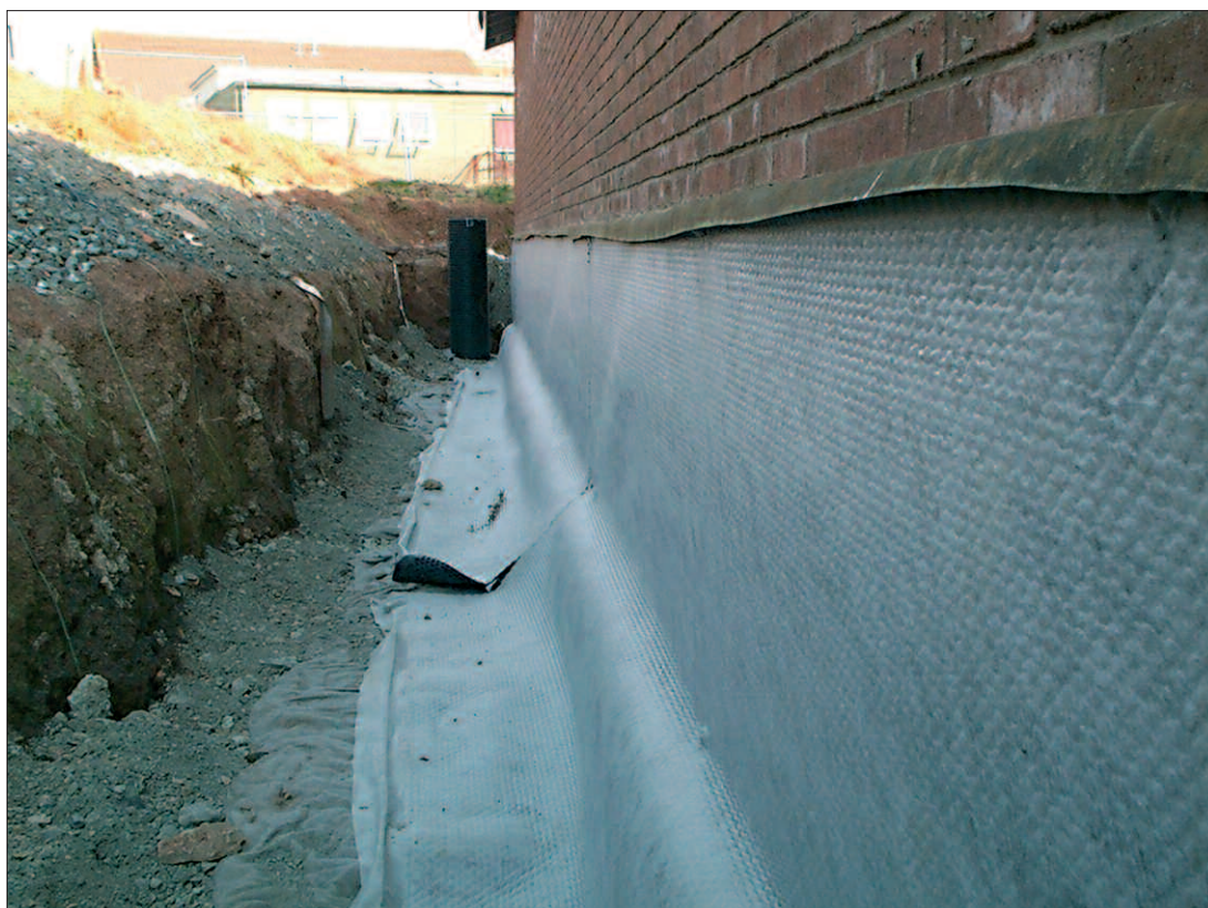
Above and left: Newton Geodrain used in new build basement.
