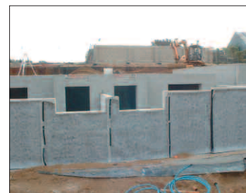
Top: Newton Geodrain used in groundworks of a sports stadium.
