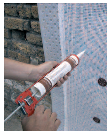
Top: Newlath 2000 used externally at Alltwn School to cure penetrating damp..
