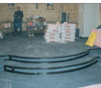
Above and right: Newton Slimline flooring membrane used in the Russian Orthodox Church in London as part of the Newton System 500.
