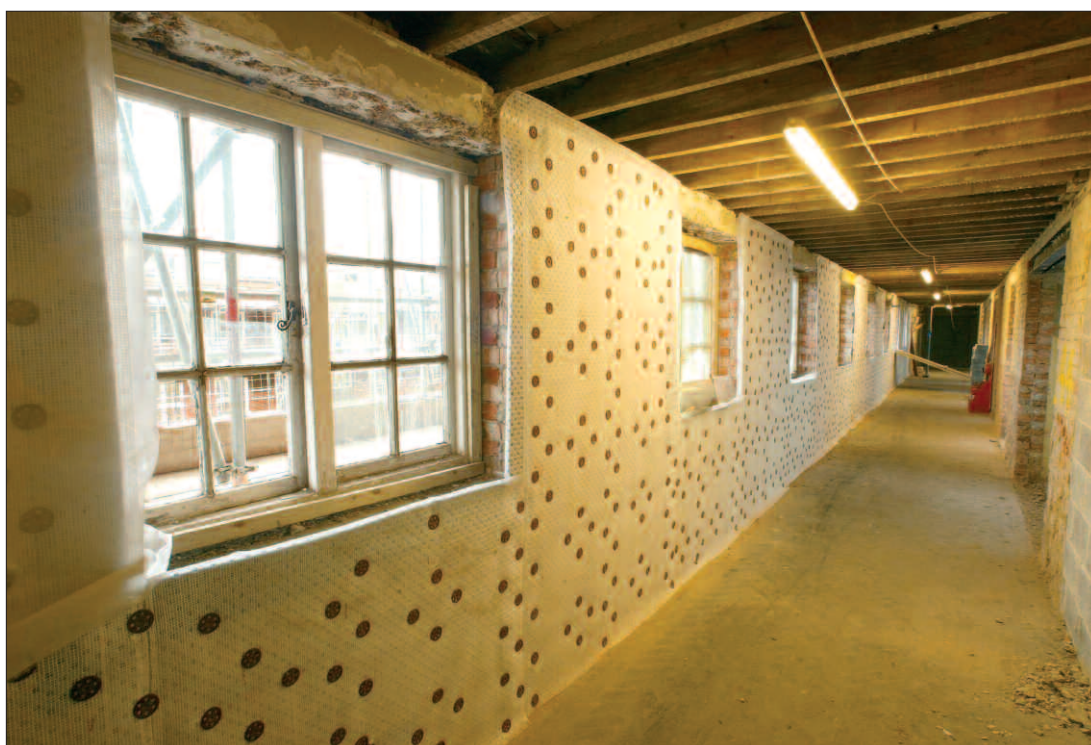
Top: Newlath 2000 used externally at Alltwn School to cure penetrating damp..
