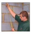
Oldroyd P can also be used on external walls to provide protection against penetrating damp.
